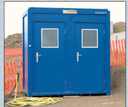
WC cabin on a building site
